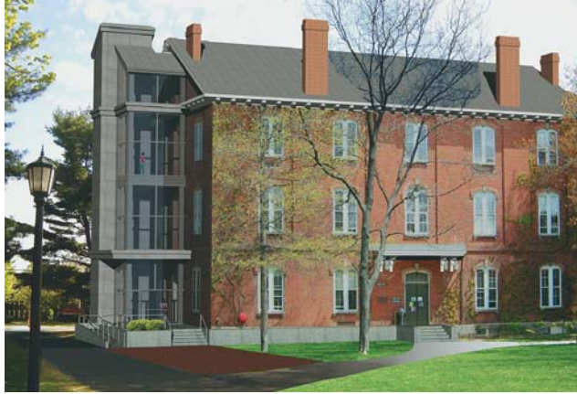
A rendering of the renovated Adams Hall, complete with its new stair tower.
