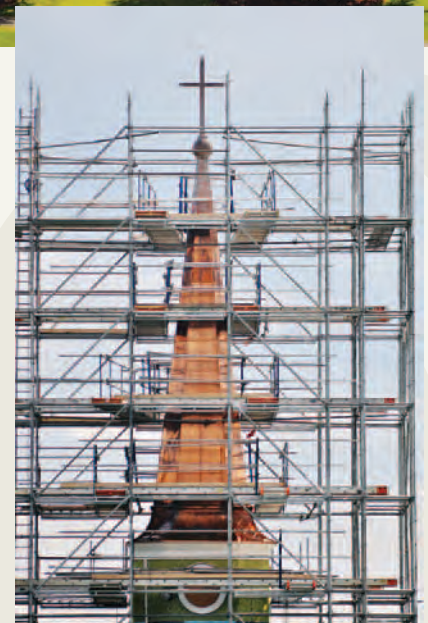
Lorimer Chapel steeple, encased in a 122-foot-high scaffolding cage during the restoration.
