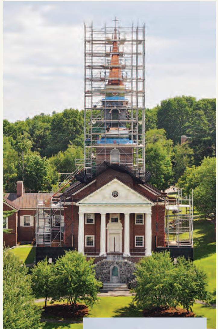
Lorimer Chapel steeple, encased in a 122-foot-high scaffolding cage during the restoration.
