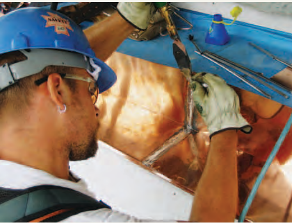
Michael Pontbraind concentrates on soldering the new copper roof.
